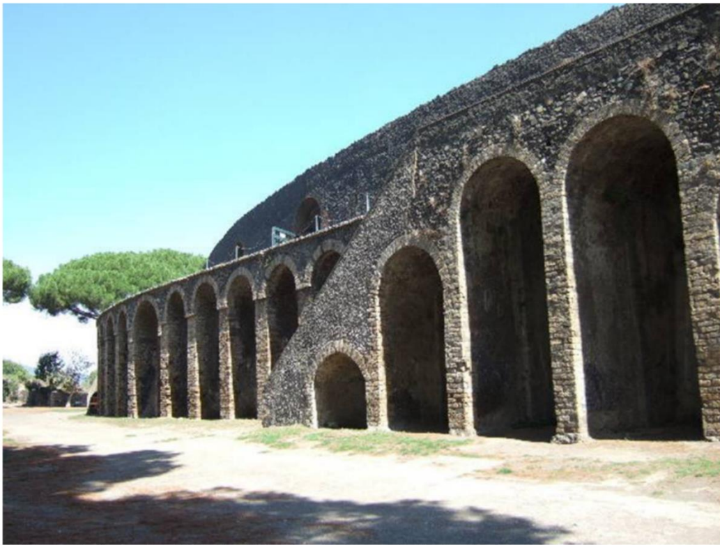
II.6 Pompeii. September 2005. Amphitheatre, central west side double staircase.
